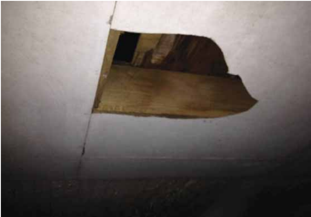
Photograph No. 7 Transite (ACM) ceiling in Dairy barns 3 and 4.
