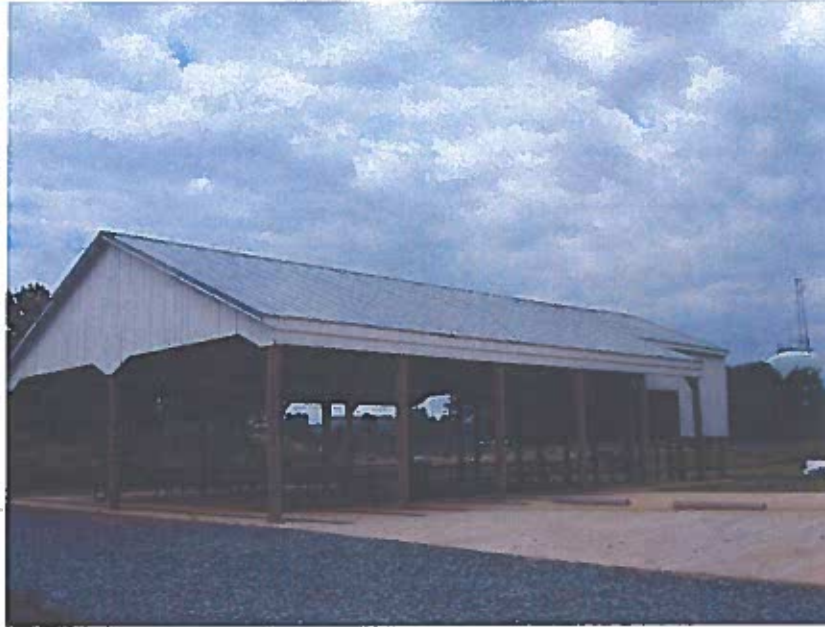
Photo 1: Overall view of building.
