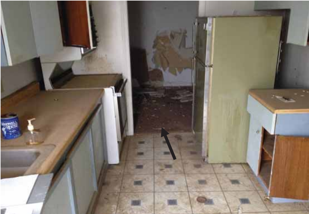
Photograph No. 6 Building 6, ACM vinyl under carpet (background)
