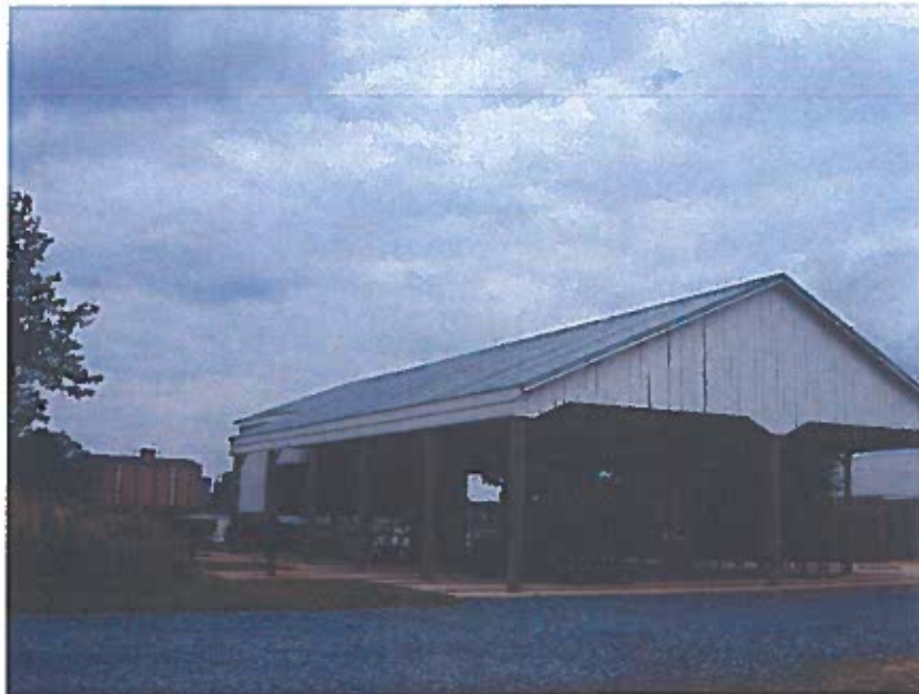
Photo 2: Overall view of building.
