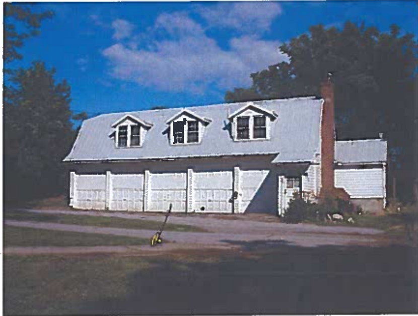
Photo 1: Overall view of building.
