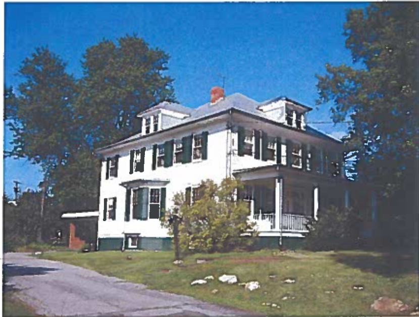
Photo 1: Overall view of building.
