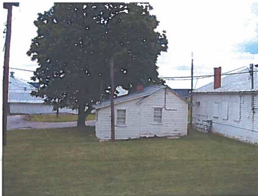
Photo 1: Overall view of building.
