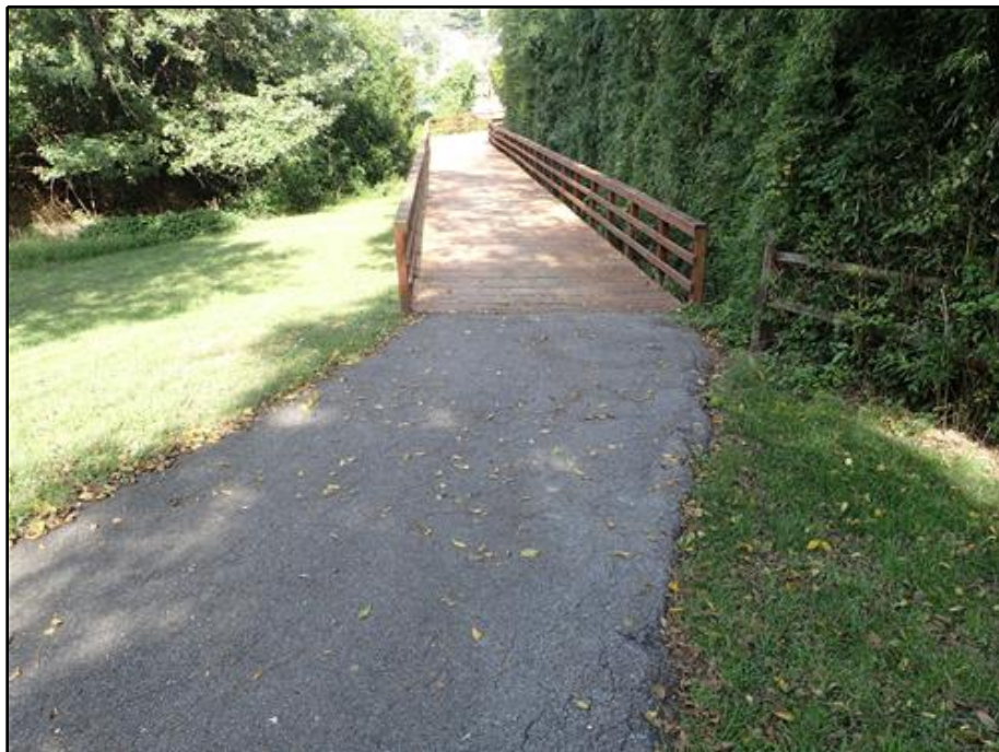
4. East Approach Looking West
