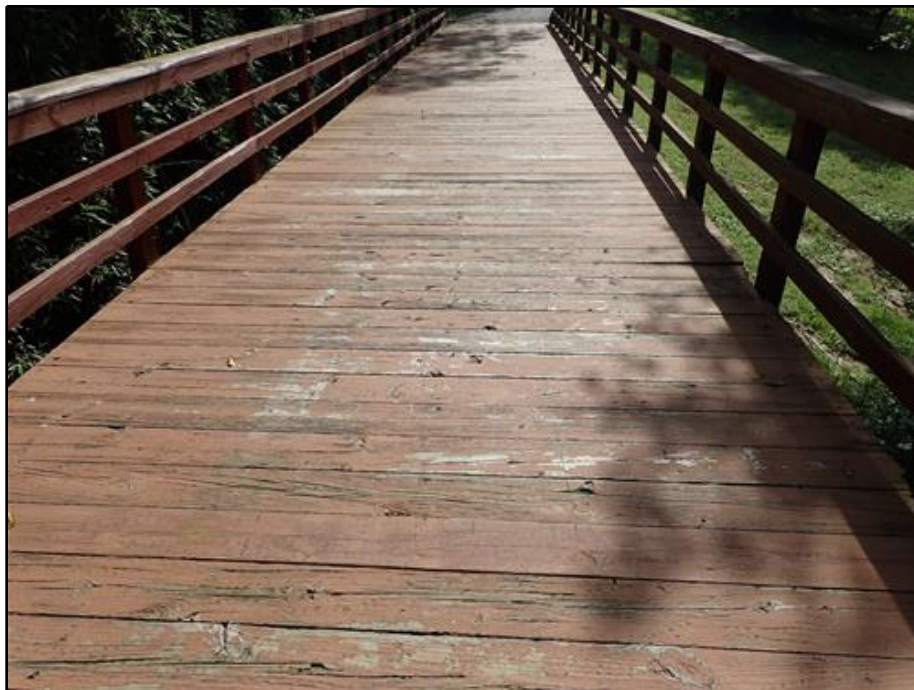
8. Overall Deck Surface
