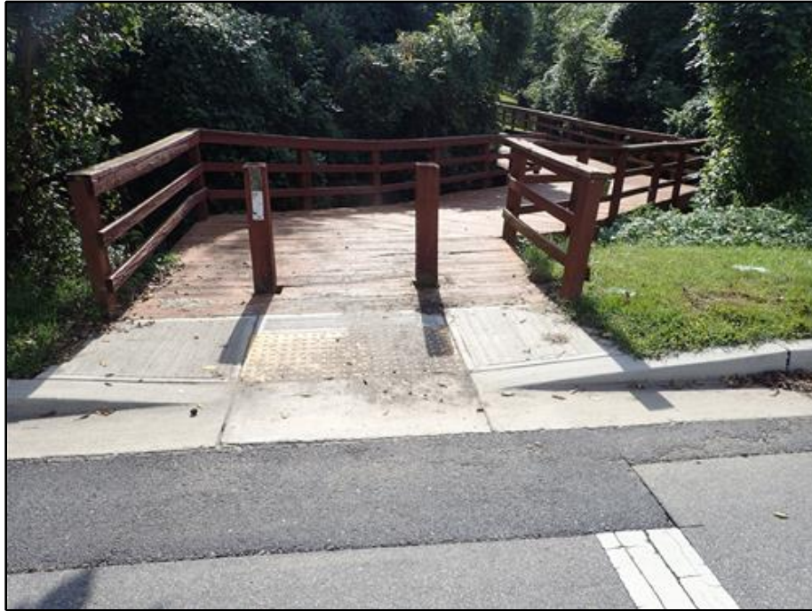
3. West Approach Looking East
