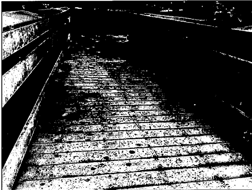
12. Main Span View of Deck Looking South
