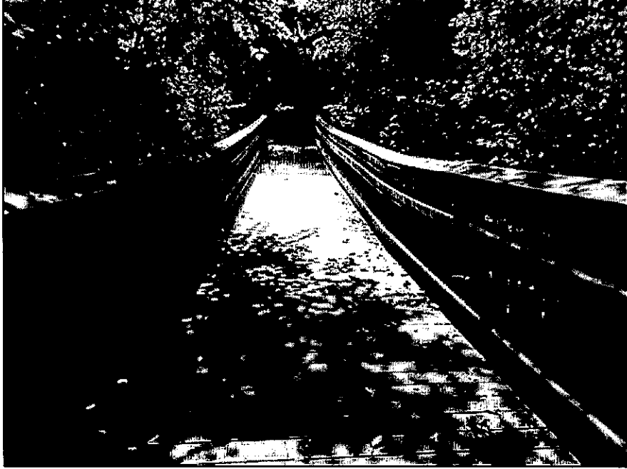
13. General Deck View Looking North
