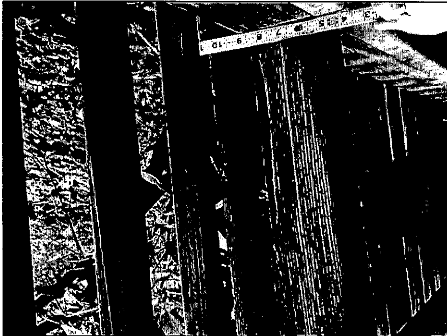
17. Up to 1 1/2" Open Split in 9th Wood Post from the South End of the East Railing
