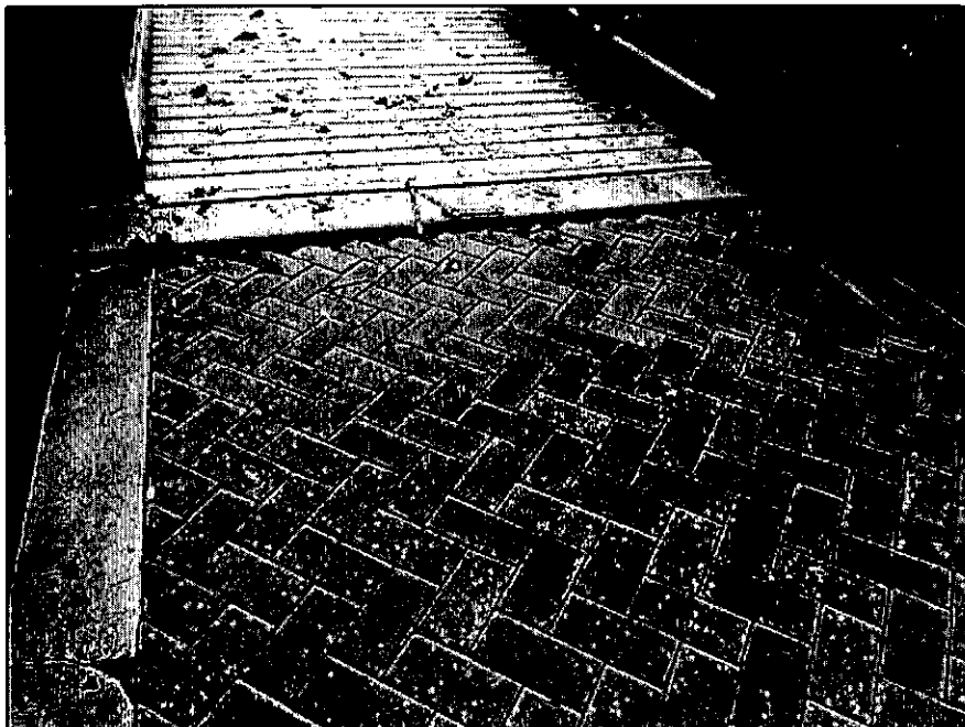
10. Up to 1 1/2" Settlement at the North Approach Concrete Backwall; Possible Trip Hazard
