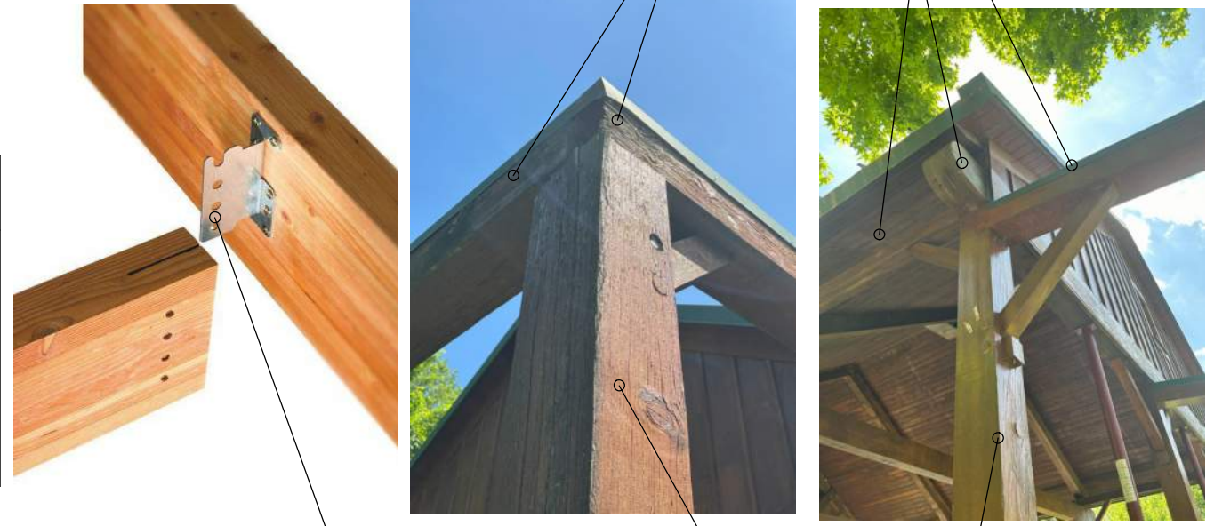
SIMPSON STRONG-TIE CJ3Z (CONCEALED IN THE BEAM)
