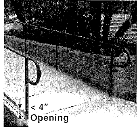
Handrail* & Wall Barrier Edges
