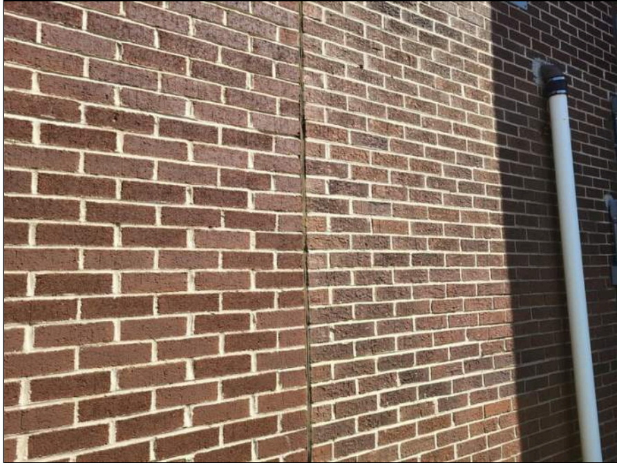
23 - Brown Wall Expansion Joint
