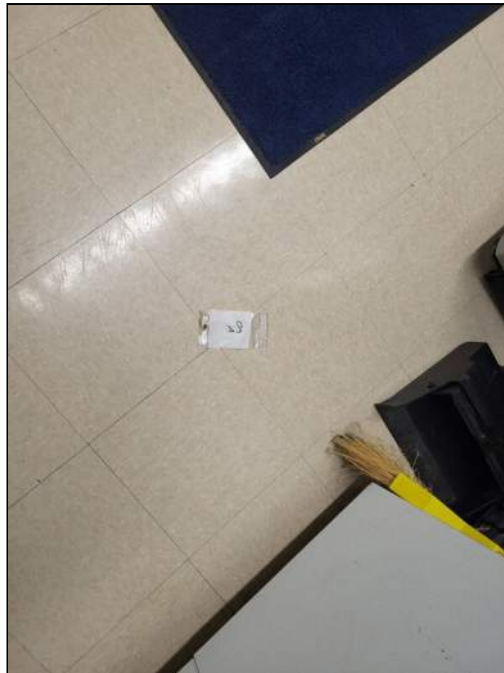
40 - 12"x12" Tan Mottled VFT with Yellow Mastic Second Layer with Black Mastic
