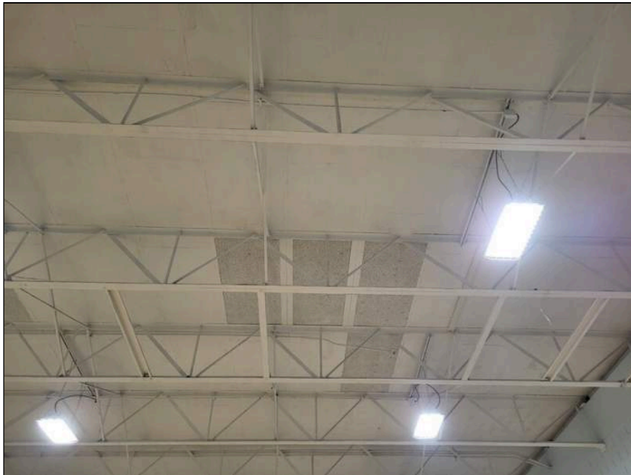
16 - Gymnasium Suspect Ceiling
