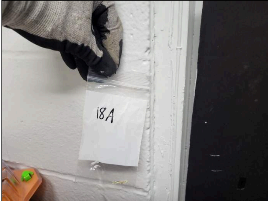
7 - White Interior Window Caulk
