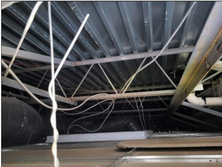
36 - Above Ceiling Plenum
