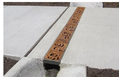
Figure 15: example of channel drain under sidewalk
