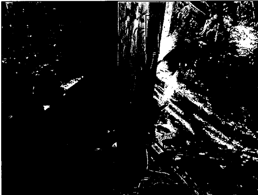
40. Bent 3, North Pile - Two (2) Areas of Decay with 1/2 in. Pick Penetrations up to 8 in. High
