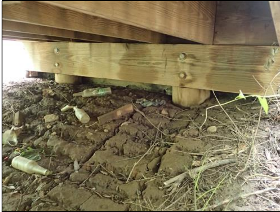
23. Overall View of North Abutment
