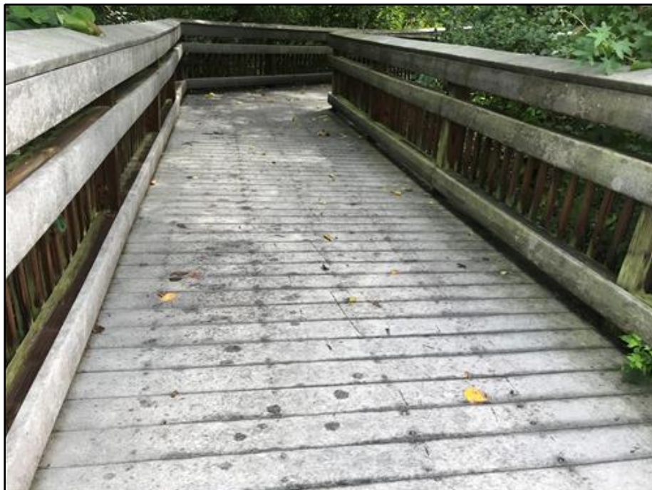
12. Main Span View of Deck Looking South
