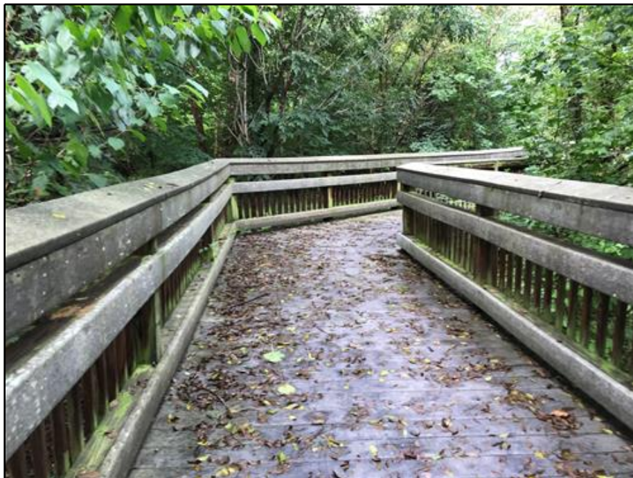
14. General View of Deck at the South end
