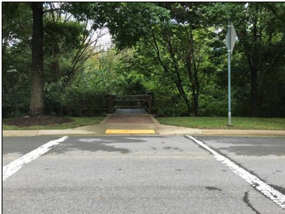
4. South Approach Looking North
