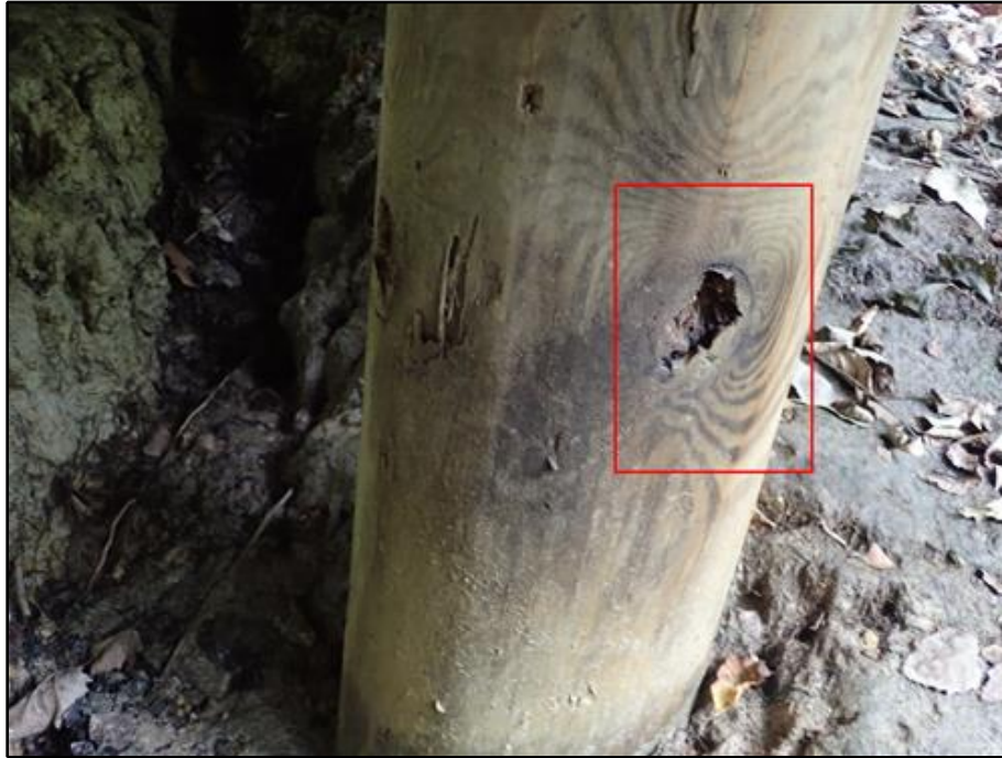
29. Approximately 3" High x 2" Wide x Up to 3/4" Pick Penetration Rot in west Pile at Bent 10
