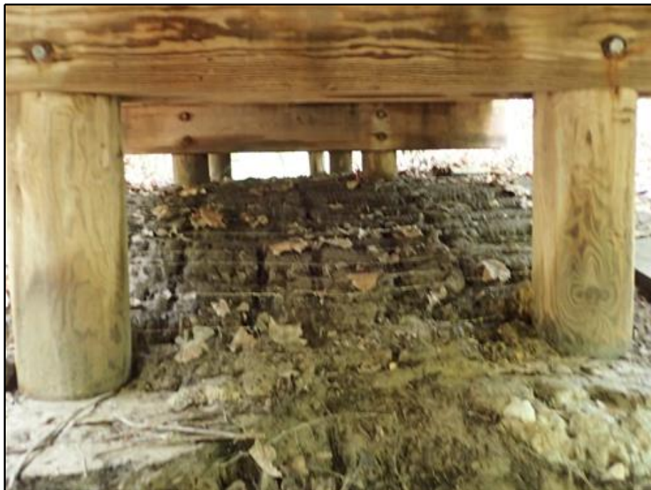
26. Typical View of Piles
