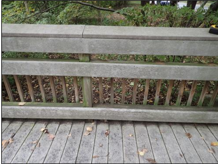
15. Typical View of Railings
