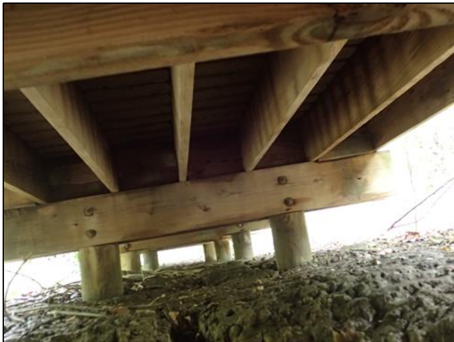
20. Typical View of Underside
