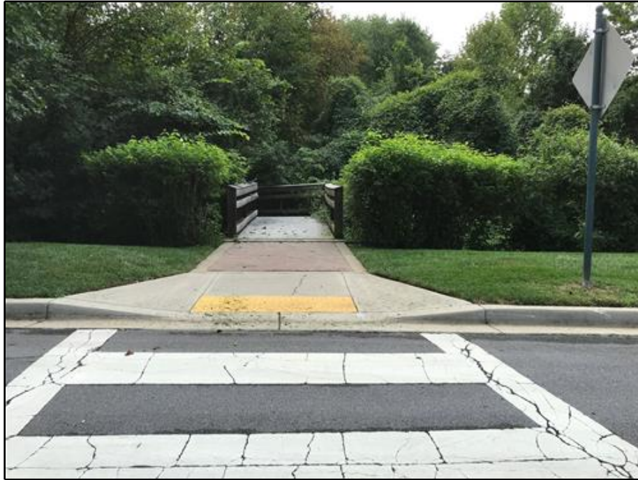
3. North Approach Looking South
