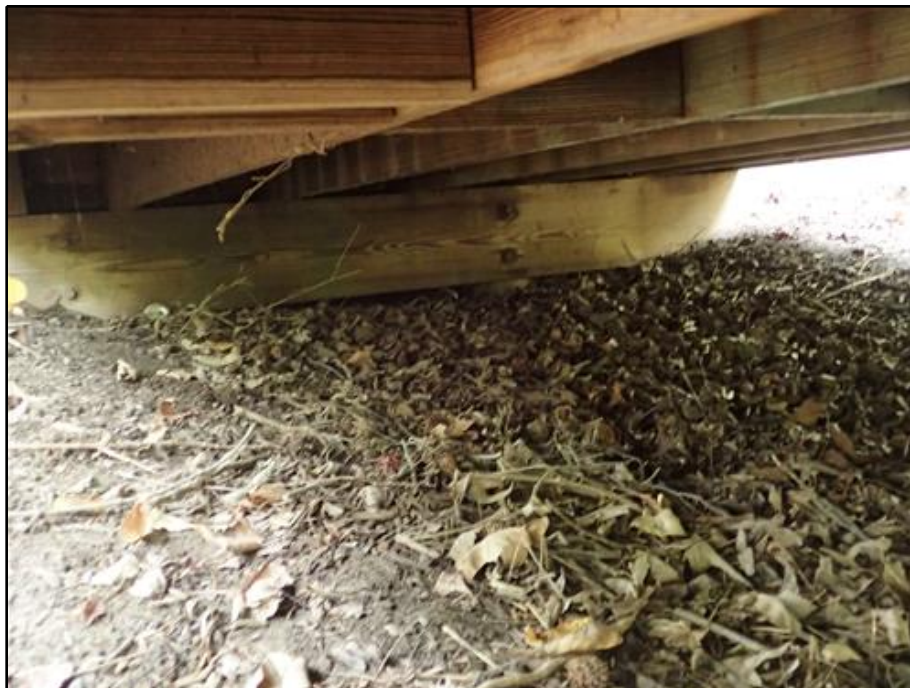
24. South Abutment View From East
