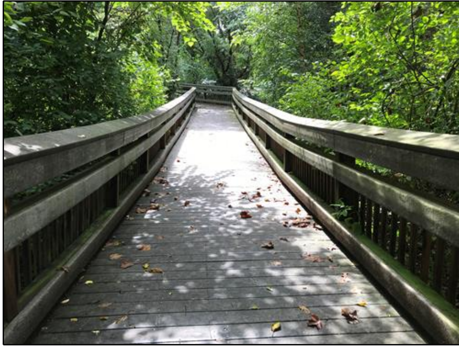
13. General Deck View Looking North
